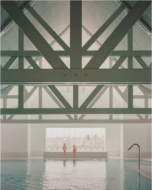
Refurbishment and extension of a community swimming pool, Saint-Méen-Le-Grand (Brittany), 2023 Photo: Charles Bouchaib
